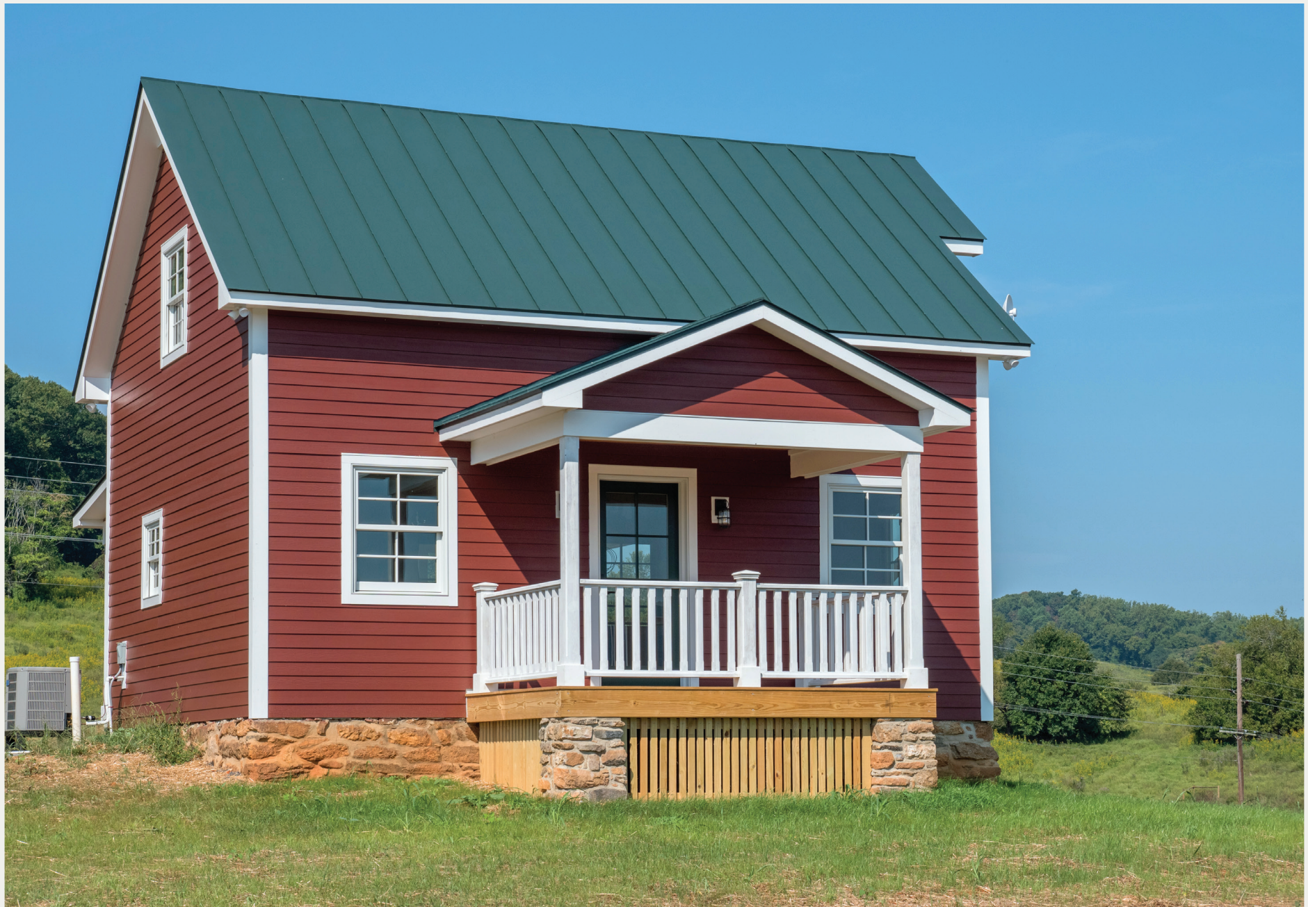
Brand new office – other than the historic foundation – at Clover Hill.
